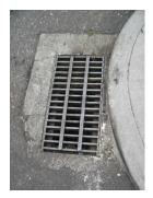
Water that falls on the street in the form of rain or water from your sprinkler or hose, enters catch basins on the street and is transported through pipes where it is discharged to a local stream. Never dump chemicals, soil, litter, oil, or any contaminant on a hard surface where it can be washed to the street. Water or contaminants that enter the stormwater system are not treated. Help keep your local streams clean and wildlife healthy.
